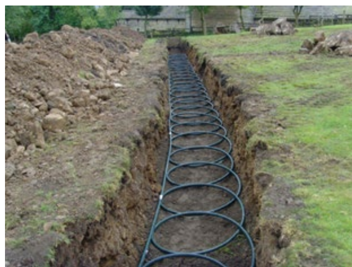
Figure 11 – Typical horizontal trenches for ground heat source
